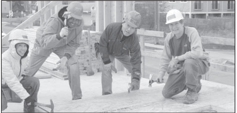
Happy hammering volunteers make headway at High Point.
