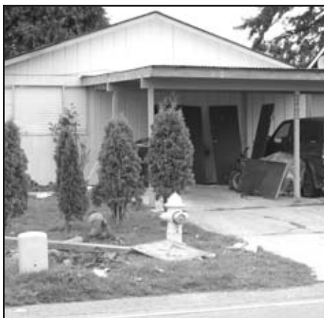
Before remodel of Westway rehab.
