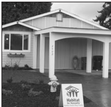
After remodel of Westway rehab.
