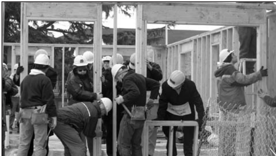
Celebrating the raising of the wall of one of the High Point duplex units during the announcement by HUD.
